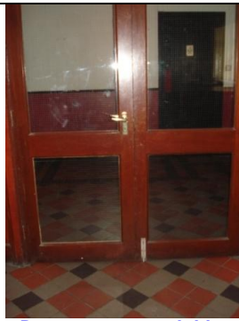
Door to entrance lobby
